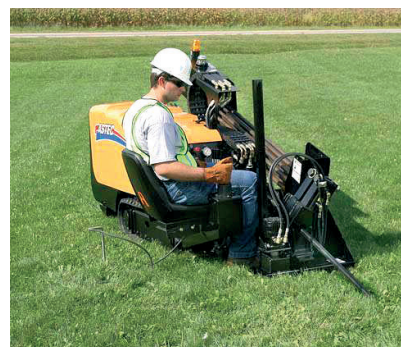
Fot. Astec Underground
