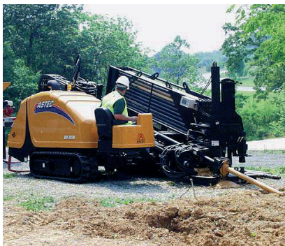
Fot. Astec Underground
