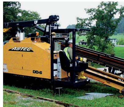
Fot. Astec Underground
